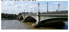
The first Battersea bridge was built of wood in 1771-2 and it replaced the regular ferry between Chelsea and Battersea. Then the only bridge between Westminster and Putney, it transformed Chelsea from a village to a small town. It was demolished in 1881 and was replaced in 1886-90 by the present bridge with 5 cast iron arches designed by Sir Joseph Bazalgette.
