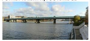
Built in 1887-9 for the London and South Western Railway with 5 spans of lattice-girder construction. It was built by William Jacomb, Brunel's assistant on the ship, the *Great Western*.
