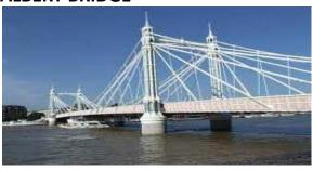
Constructed on a straight link suspension system in 1871-3 and built as a cantilever structure, each half supported by its straight wrought iron bars radiating from the top of the highly ornamental cast iron towers. The side girders of the parapets were hung from vertical steel suspenders. Thus it was a hybrid type of bridge containing elements of both cantilever and suspension. In 1971-73 the deck was strengthened to take increased traffic loads.
