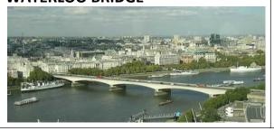
The first bridge was opened by the Prince Regent on the second anniversary of the Battle of Waterloo. Made of granite, it was originially known as the Strand Bridge. It was demolished in 1936 due to subsidence and replaced by the present bridge. The arches were clad in Portland stone from the South West of England; the stone cleans itself whenever it rains.
