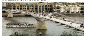
The flat steel suspension bridge carries pedestrians over the river between Tate Modern and St Paul's Cathedral. Also known as the 'Wobbly Bridge' because of the swaying that occurred at its official opening in 2000. The bridge was closed while the problem was solved using a system of dampers.
