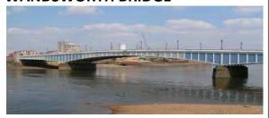
The first Wandsworth bridge was built by J.H. Tolmé in 1870-73. It was a continuous lattice-girder bridge of 5 spans. It was freed from tolls in 1880. In 1936-40 it was replaced by the present 3 spanned bridge of steel-plate girder cantilever construction, designed by Sir Pierson Frank, (elected president of the Institution of civil Engineers 1945 to November 1946)
